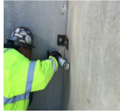
STEP 2: INSTALL SPRAY FOAM INSULATION IN JOINT
