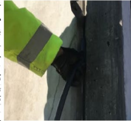
STEP 1: INSTALL BACKER ROD IN JOINT
